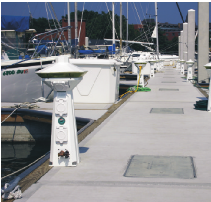
Above: Hatteras Light Power Pedestals
