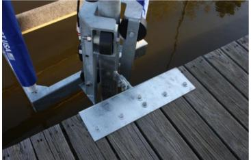
Your PWC Lift is supplied with 1 dock mount plate. Install the dock mount plate first on the dock. Remember to leave room for your lift to rotate on either side. We recommend ant least 5 ft. It is recommended to use the 4 x 1/2" bolts supplied and back them up with washers. We do not recommend lag bolting the 4 outside points. The two larger center points can be lag bolted using the larger bolts supplied.
